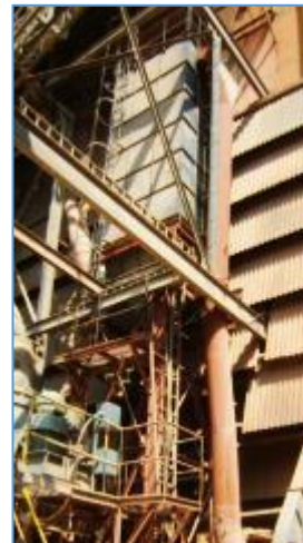
Bag filters at various material transfer points & silo top
