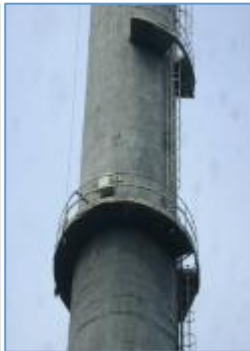
CEMS analyzers at Stacks, Cooler, CPP & Kiln stacks
